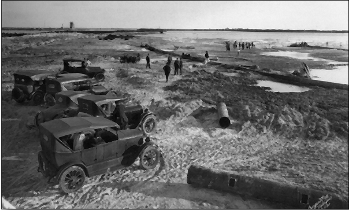
Another view of the dredging operation shows a crowd of smartly dressed visitors who arrived by car. Motorcycles can be seen at the center. Moms and Dads in suits and hats -- and even children running in the sand -- appear to be scouting locations for their new dream homes. This view was taken looking southwest.
