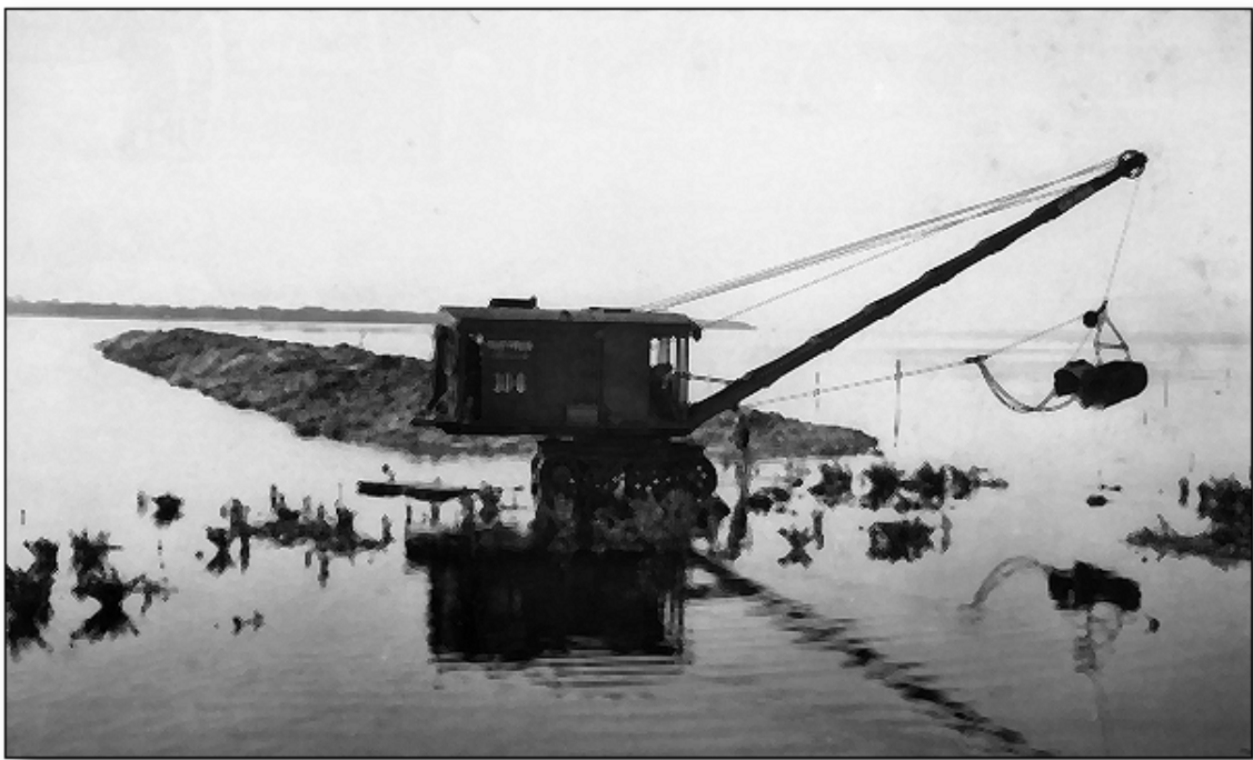
Cranes were employed along with the dredging to reposition the fill and raise the height to levels suitable for building. This scene may show the creation of connections from island to island.
